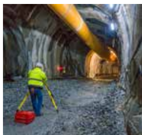
A member of Hellas Gold's survey team measures underground progress at Skouries.
