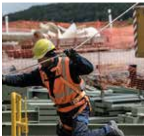
Construction at Skouries.
