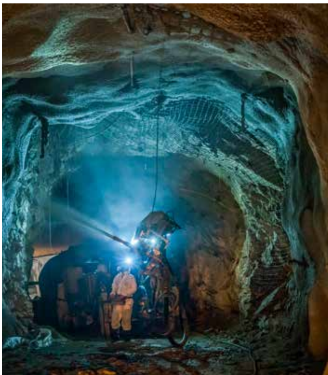
Backfilling areas at Olympias underground.
