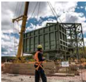
Construction at Skouries.
