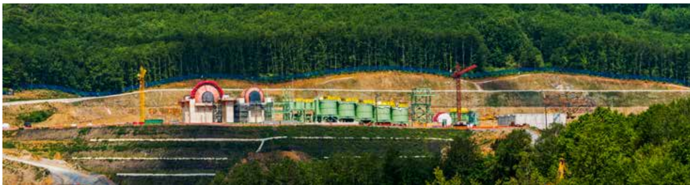
Plant construction at Skouries.
