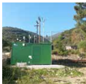
Air quality monitoring station, part of Hellas Gold's Environmental Monitoring System.
