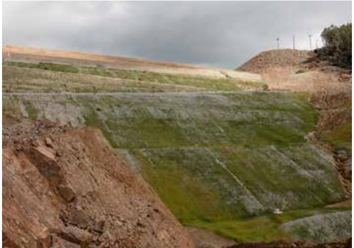
Hydro-seeding at the Kokkinolakkas Tailings Management Facility.
